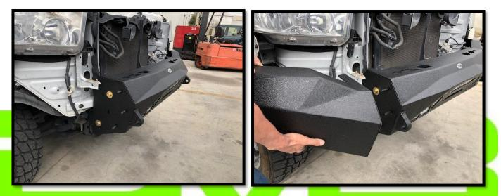
6. Once all pieces are on, with help, align the bumper with body lines and starting with the frame mounted pieces, tighten all components.
